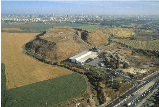
Fig. 4. Hiriya landfill, 2002. Source: Dan Region Association of Towns
