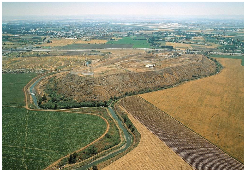
Fig. 1. Hiriya landfill, 2004. Source: Dan Region Association of Towns.
