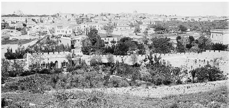
Plate 36: ACPD, General view from the Hill towards west. c.1910.
