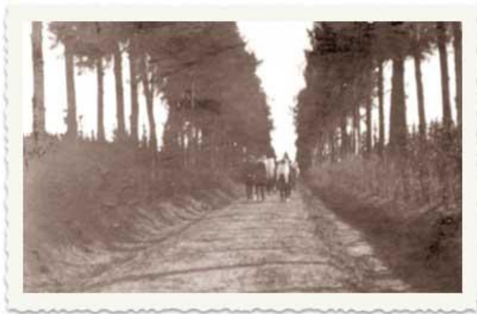
Figure 62 - Hedgerow of tall trees- Perhaps Grevillea- note drainage-irrigation furrows c. 1910
