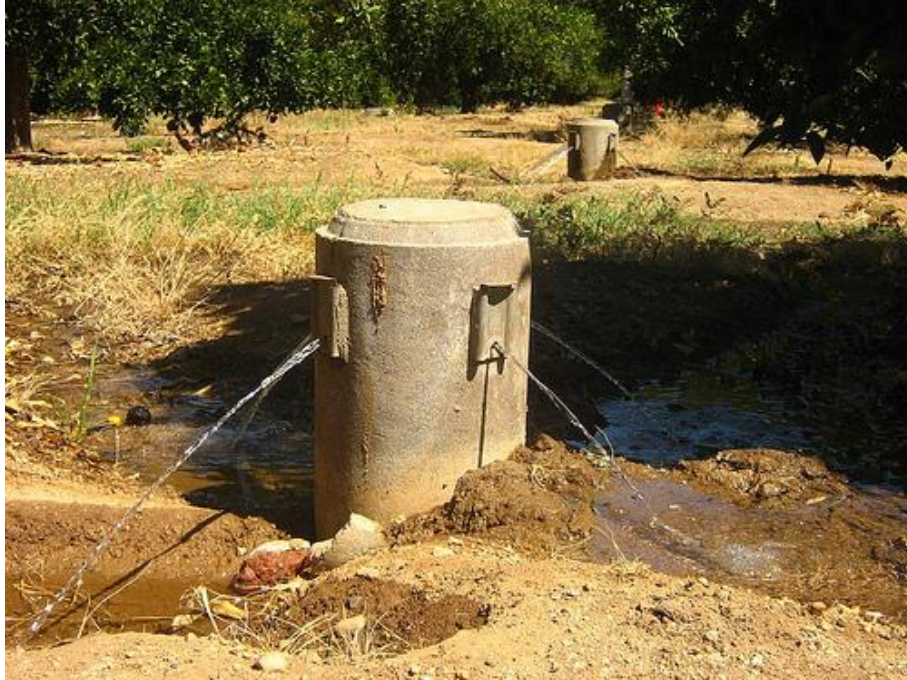
Figure 11 - The "California Irrigation System" introduced in Palestine 1936 "Yakhin Groves" using furrowed basins with water delivered by underground tubes.
