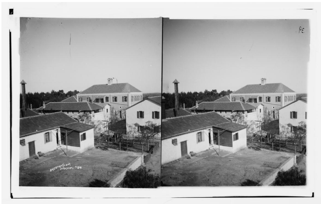
Figure 33 - Mikveh Buildings – Flower house – two levels and Synagogue c. 1920 Matson Photo service
