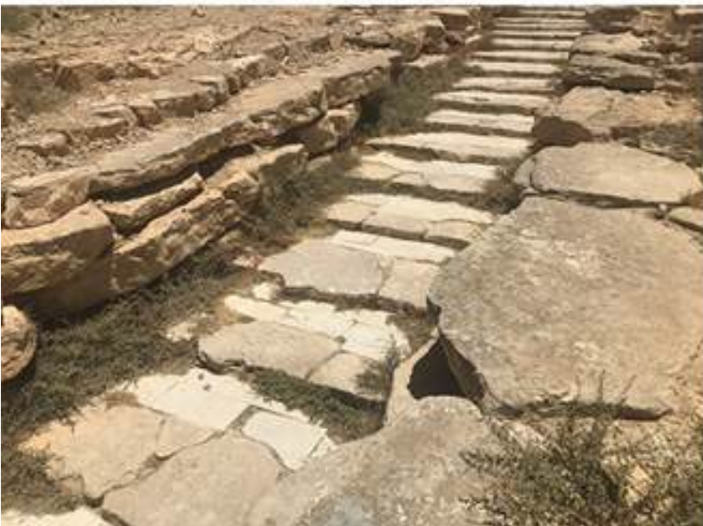
[159-61] The Albert promenade today. Top: The lookout pavillion at one entrance. Middle: View of the stone wall along the edge of the cliff. Bottom: Entrance stairs made of local stones in different cuts. Photos by author.
