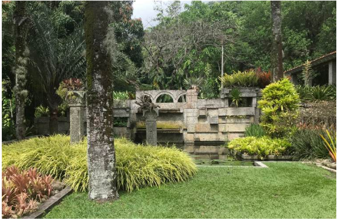
[121] Roberto Burle Marx, Retaining wall built from leftovers of a demolished historical building in central Rio, Sítio, 2019. Photo by the author.
