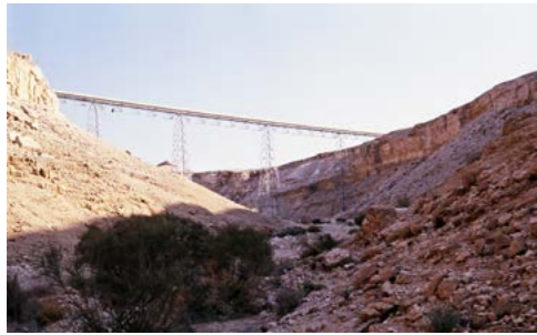
Fig. 51. The Potash conveyor belt
