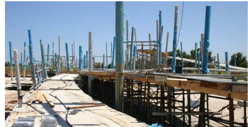
Fig. 185. The system of ramps and supporting columns under construction
