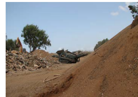
Fig. 219. Construction waste recycled on-site for re-use as subbase material
