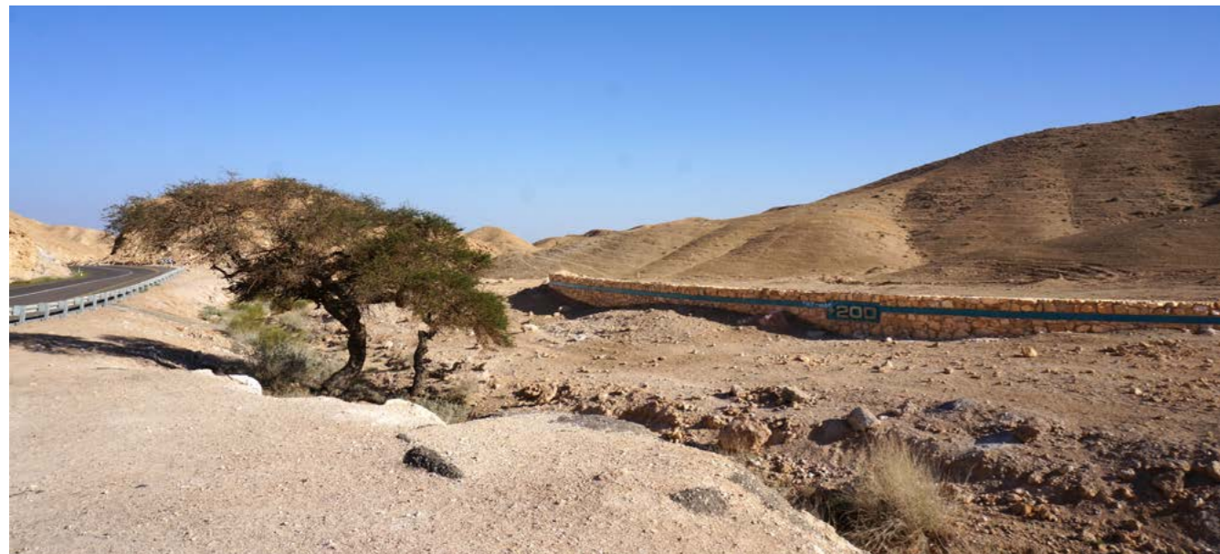
Fig. 67. The -200m contour line wall along the road from Arad to the Dead Sea
