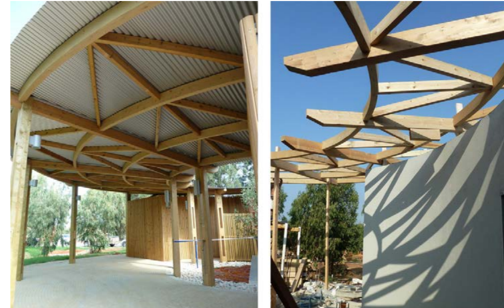
Fig. 224. The coffee shop under construction
