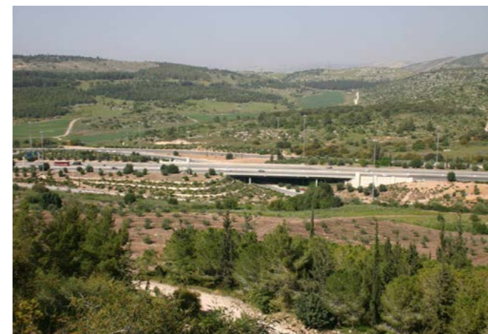
Fig. 164. View towards the interchange as seen from the higher surroundings to the east, 1996
